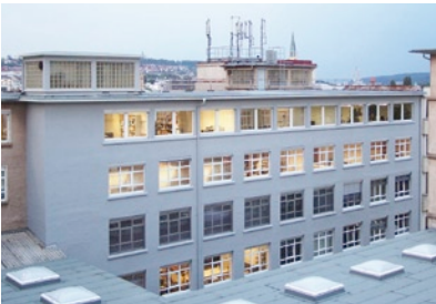
Berthold Detection Systems GmbH in Pforzheim, Germany
